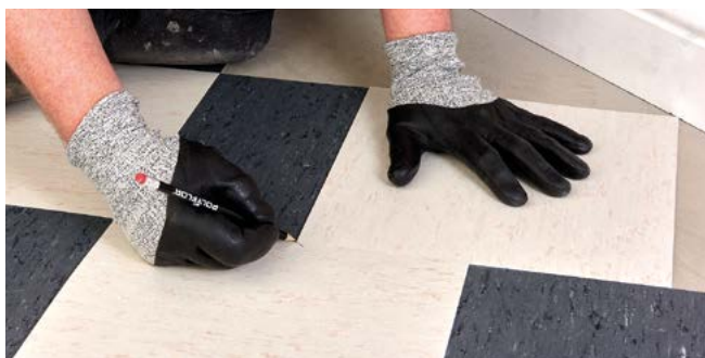
Figure 7 Marking the perimeter tiles (diagonal cut)
