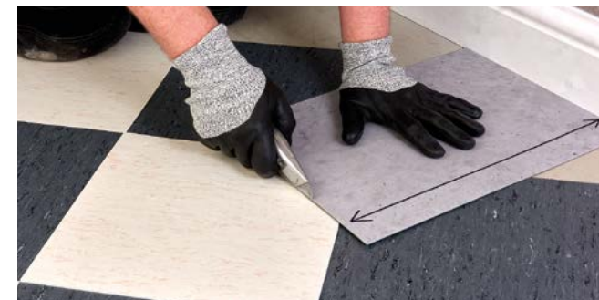
Figure 8 Cutting the perimeter tiles (diagonal cut)
